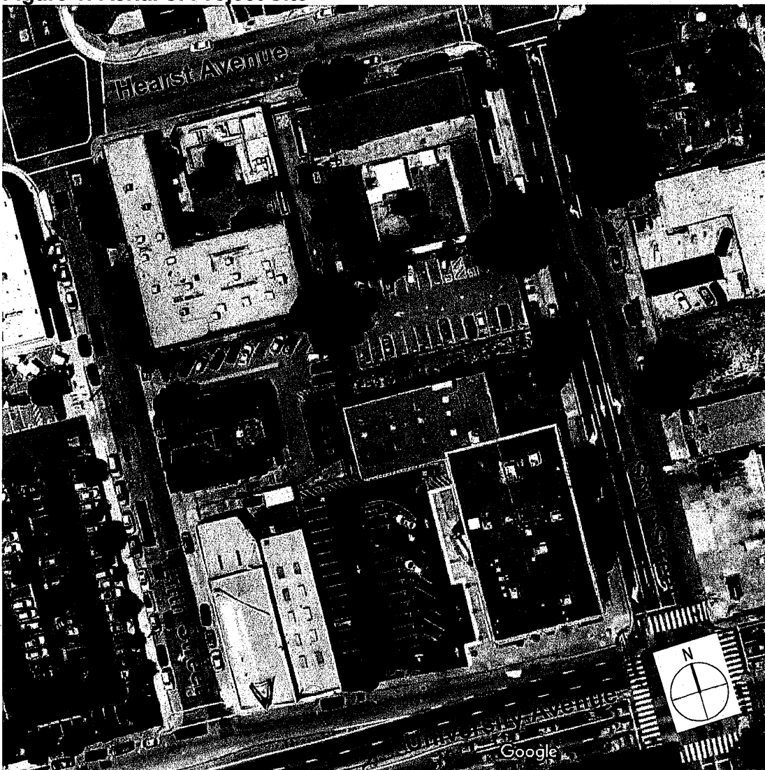
Figure 1: Aerial of Project Site
